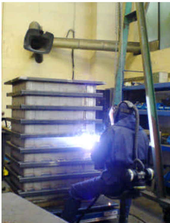
Tubular re-enforcement members being welded to an air-cooled 700L Rectangular Section Chamber under PD5500 coding
